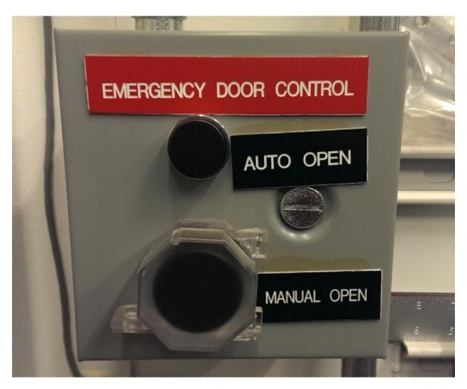
Example of a Typical Pneumatic Door Control Box Inside an Instrument Station
